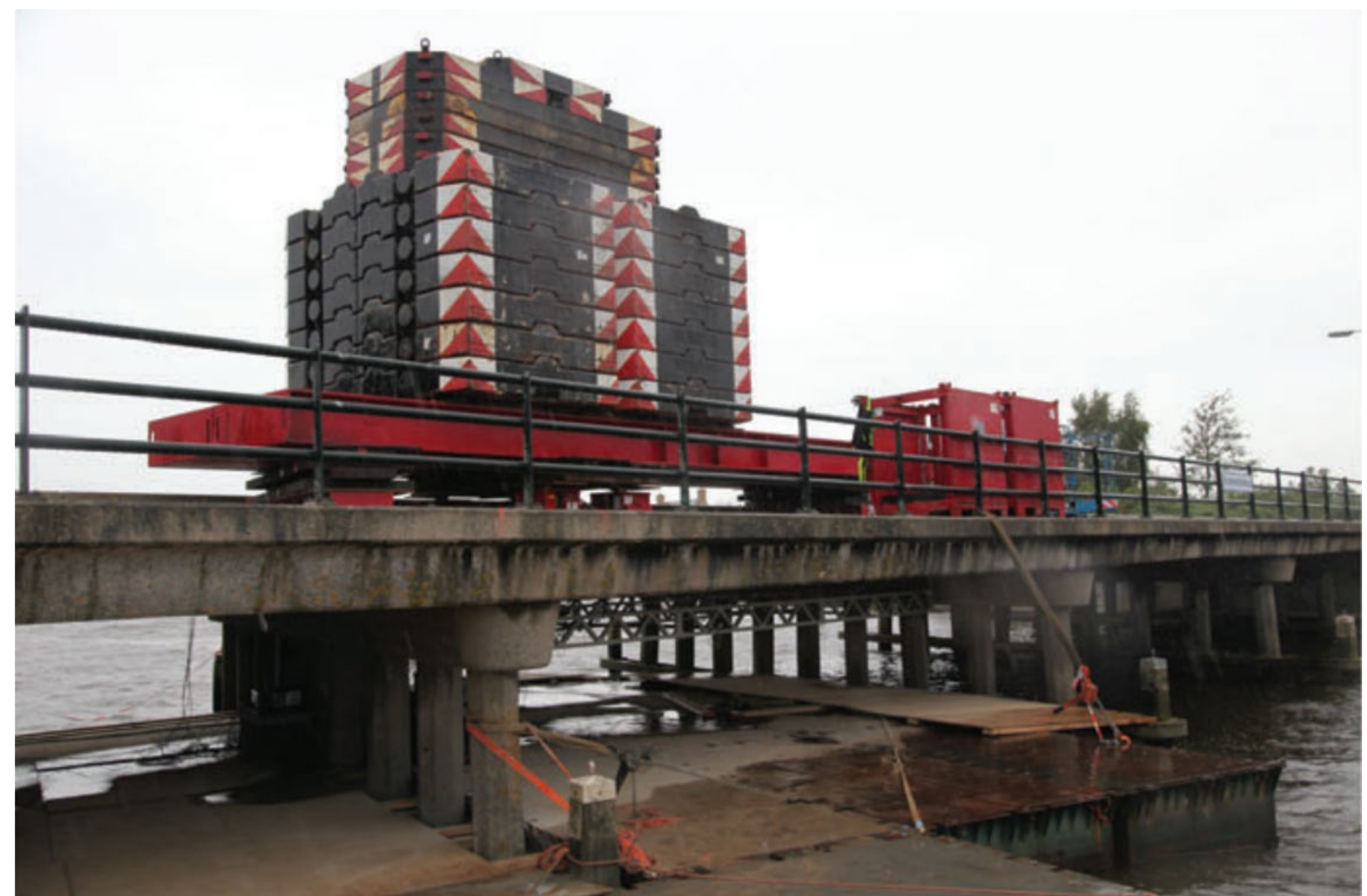
Load test on Ruytenschildt bridge using a steel load spreader structure, hydraulic jacks and counter weights
