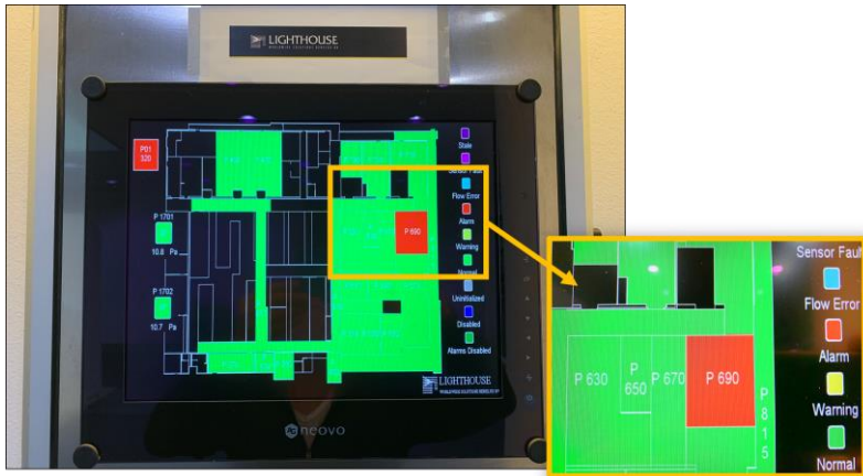
example of conditions that are out-of-spec for room P.00.69
