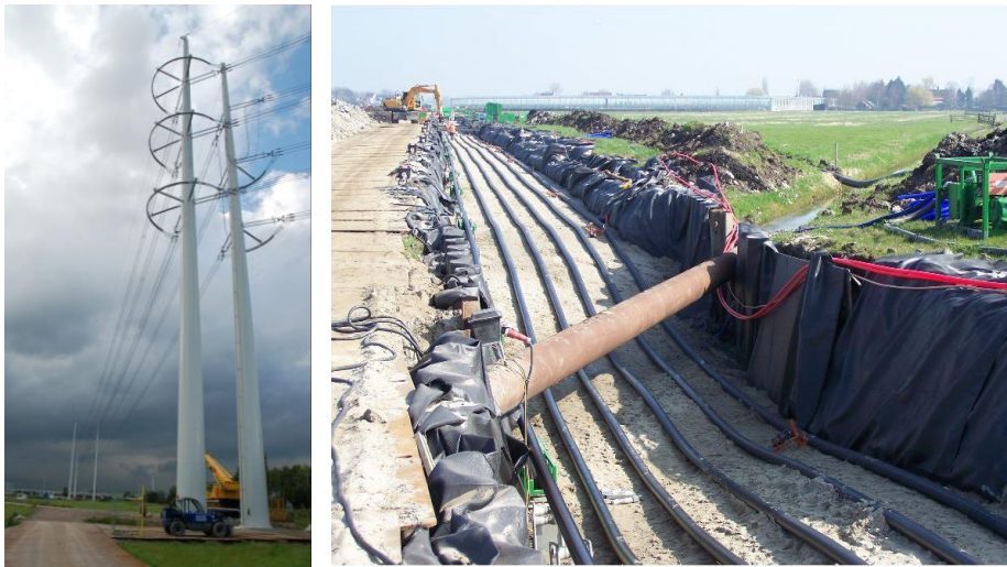
TenneT, 380kV Transmission line and cable
